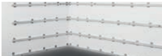
Timber battens straight onto wall
