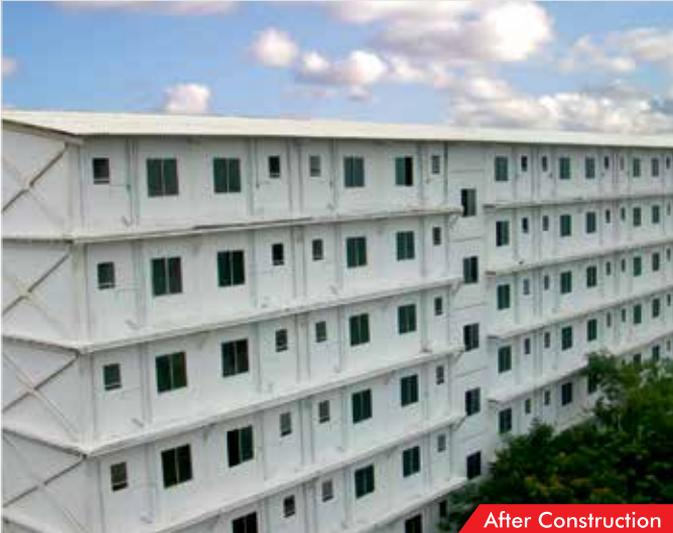
**Pre-engineered Rehabilitation Unit - External and Internal Wall**
